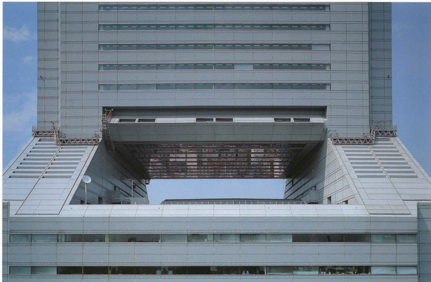
開口部 Opening penetrating of the building.
