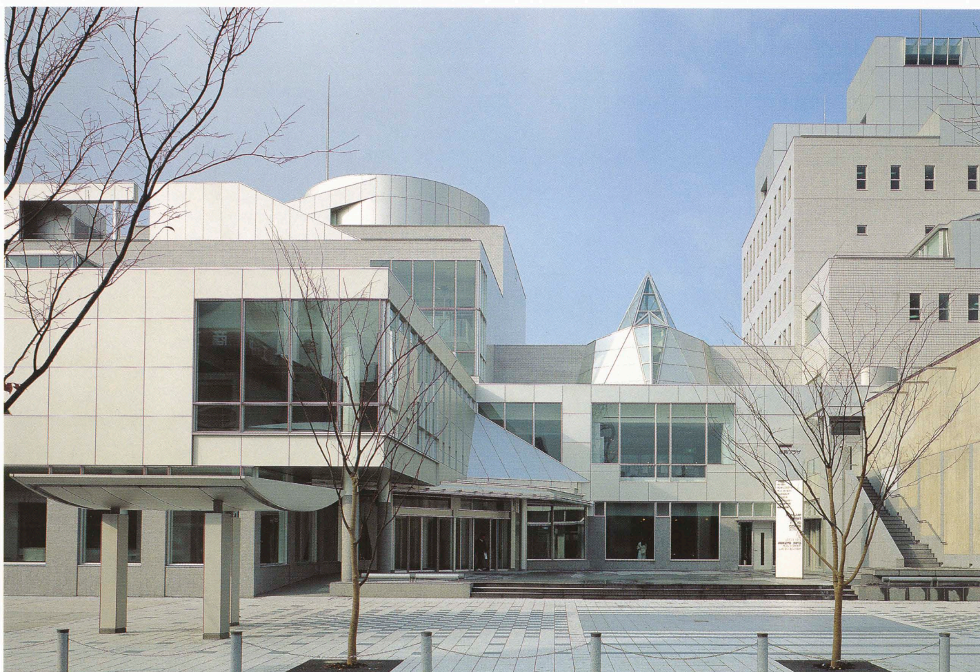
東側外観 View of the east side.
