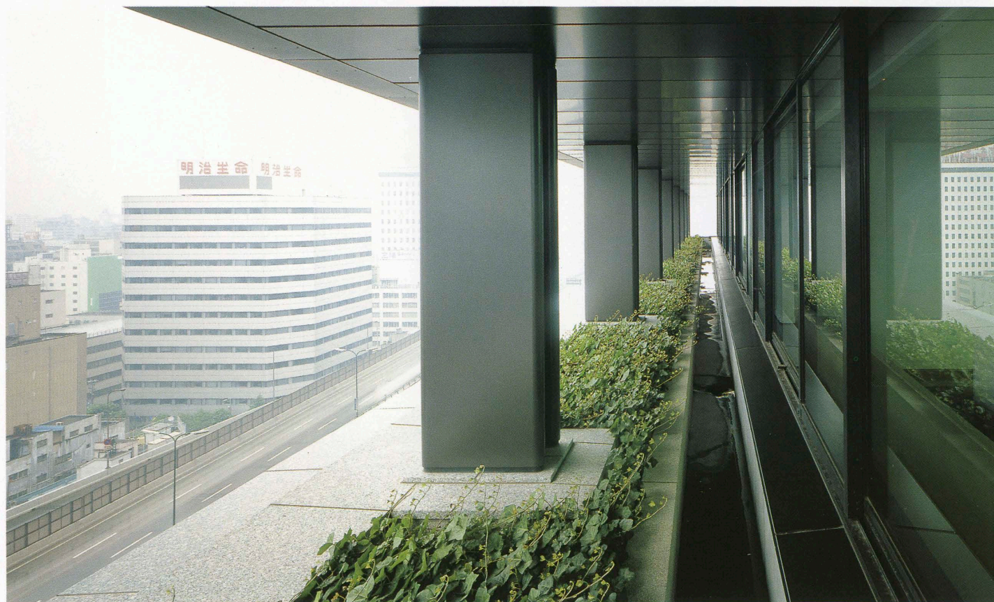
14階バルコニー Balcony on the 14th floor.
