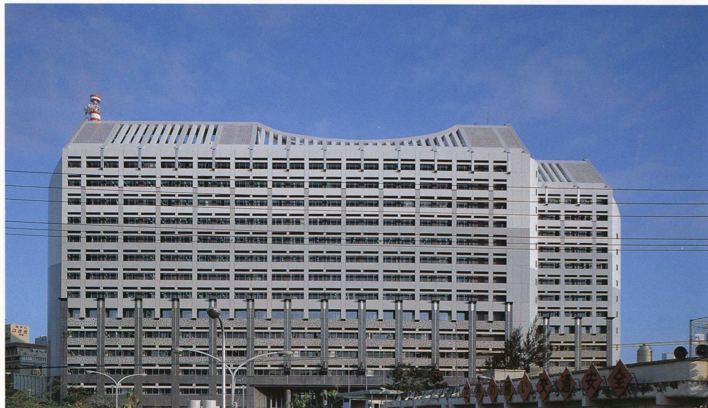
北側外観 View of the north side.
