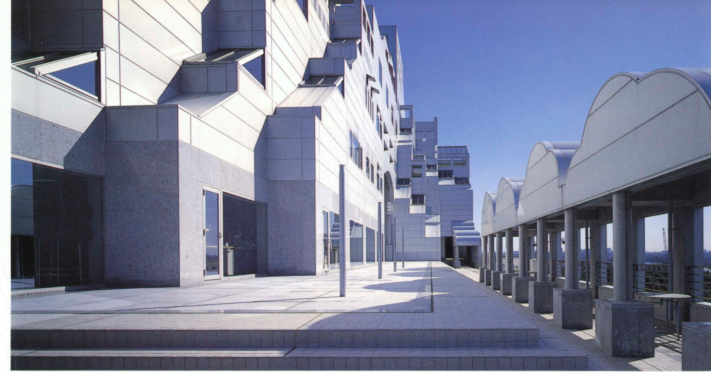
4階屋上 4th-floor rooftop area.
