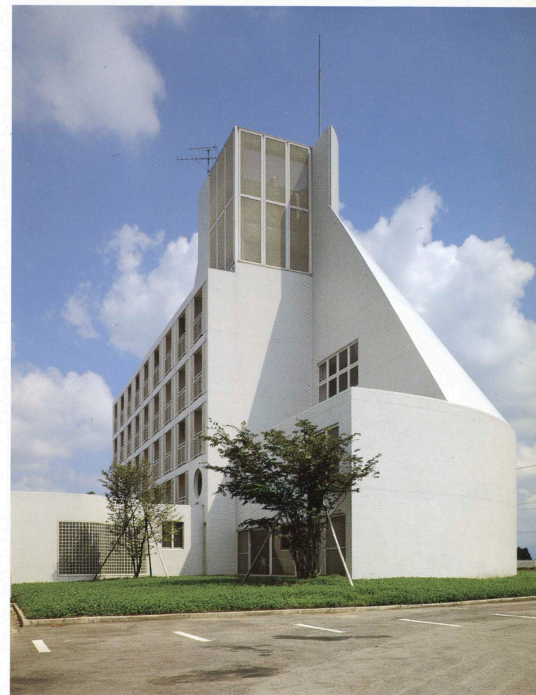
厚生施設棟北側全景 North side of welfare facilities building.
