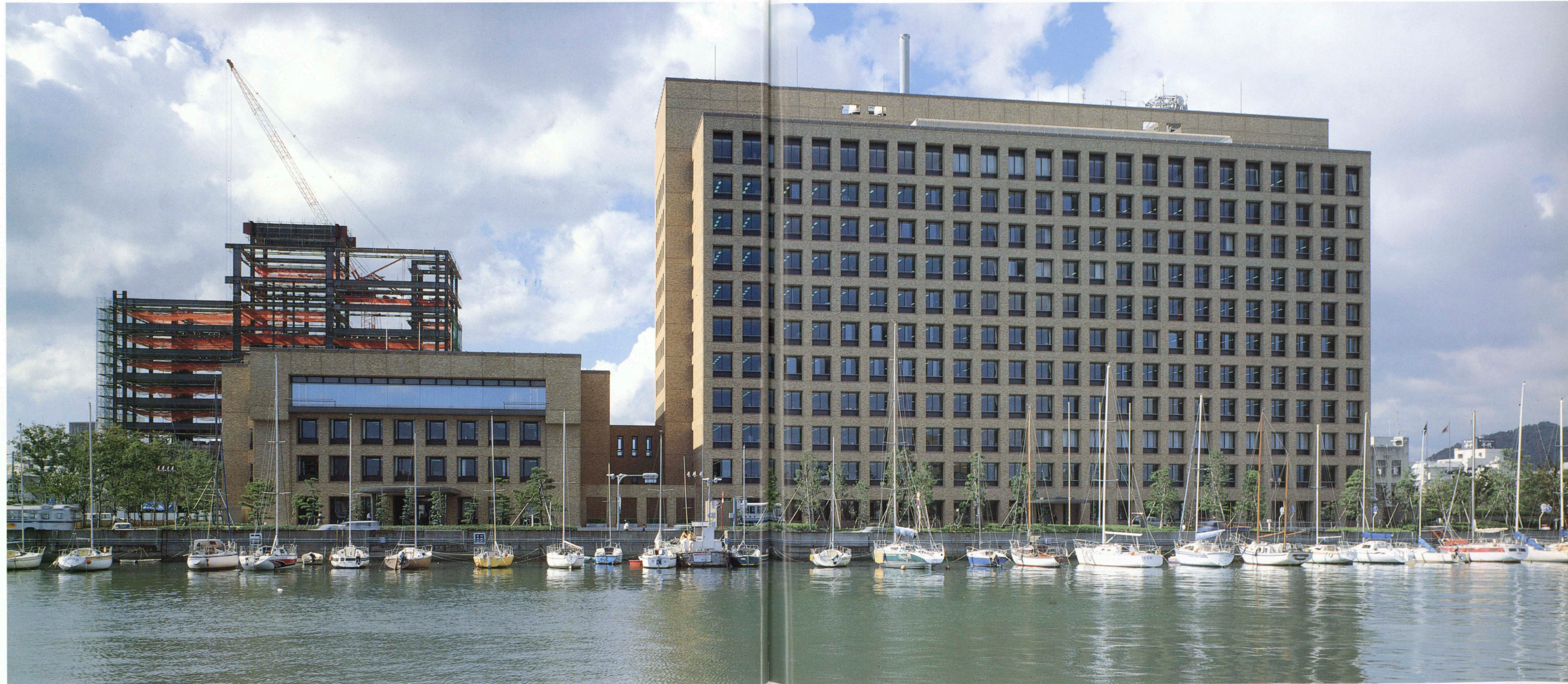
北側全景 General view from the north.
