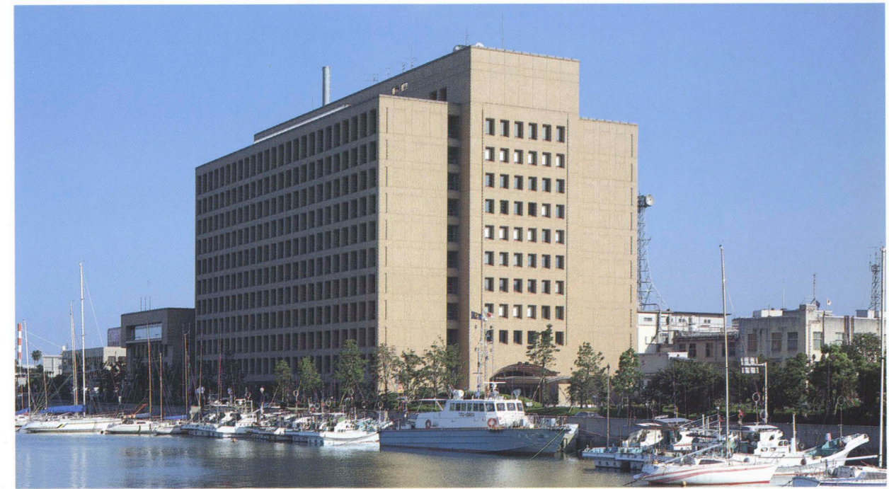
行政庁舎西側全景 General view of the administrative offices building seen from the west.
