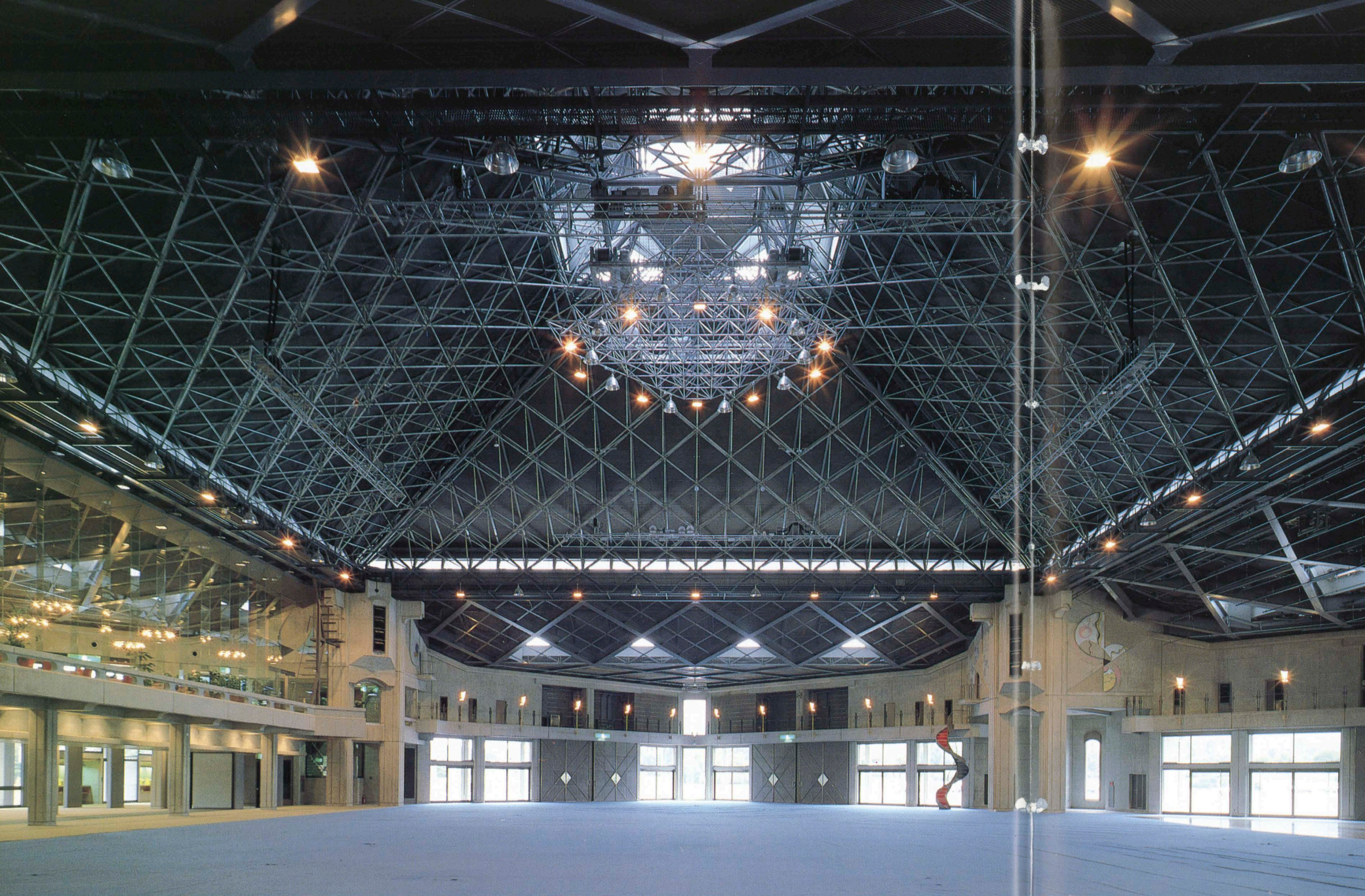
展示ホール／大屋根の立体トラスの設計は木村俊彦 Exhibition hall. The space truss of the roof was designed by Toshihiko Kimura.
