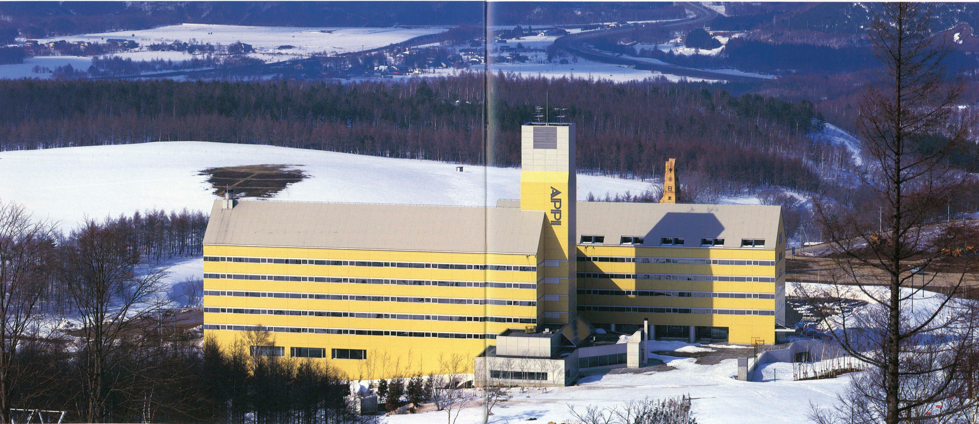
南側全景 General view from the south.
