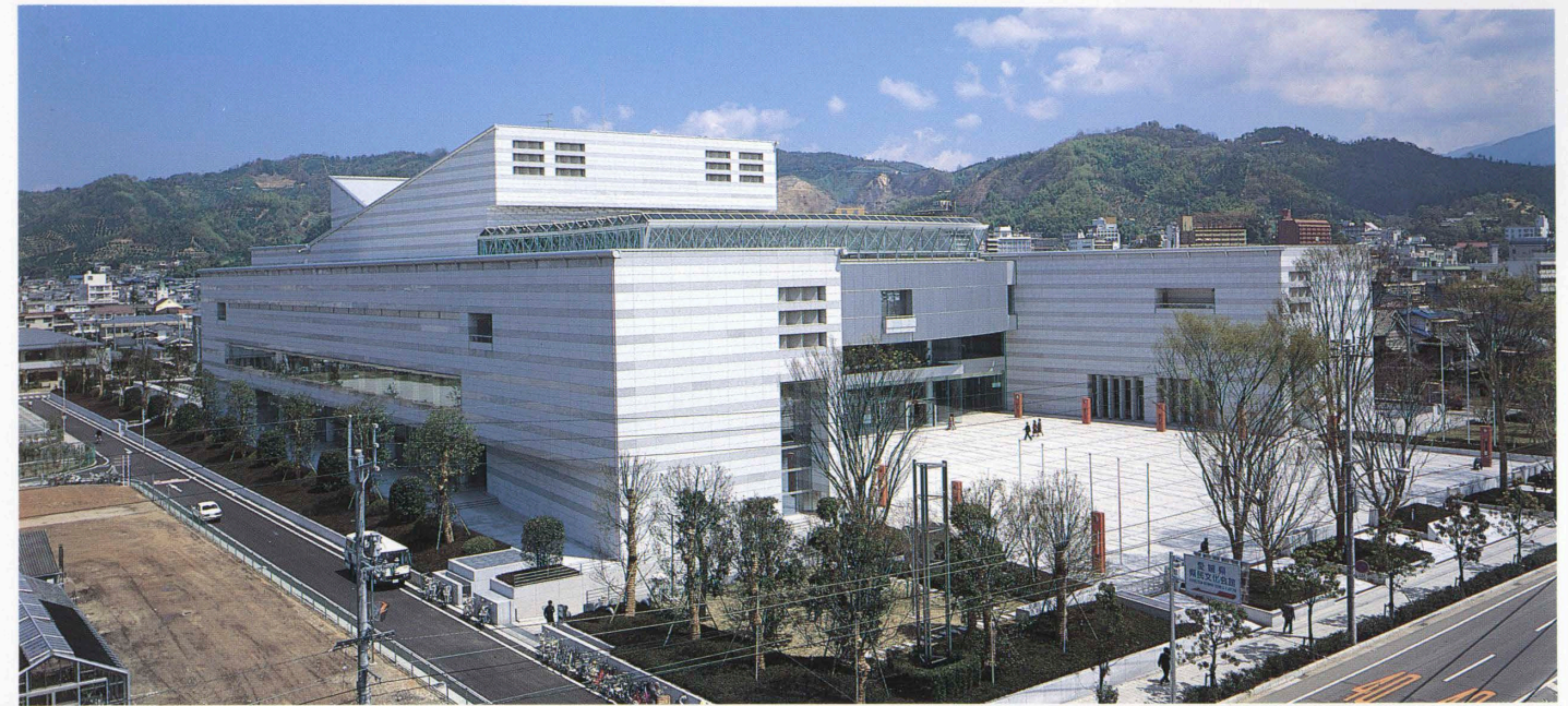
南西よりの全景 General view from the southwest.
