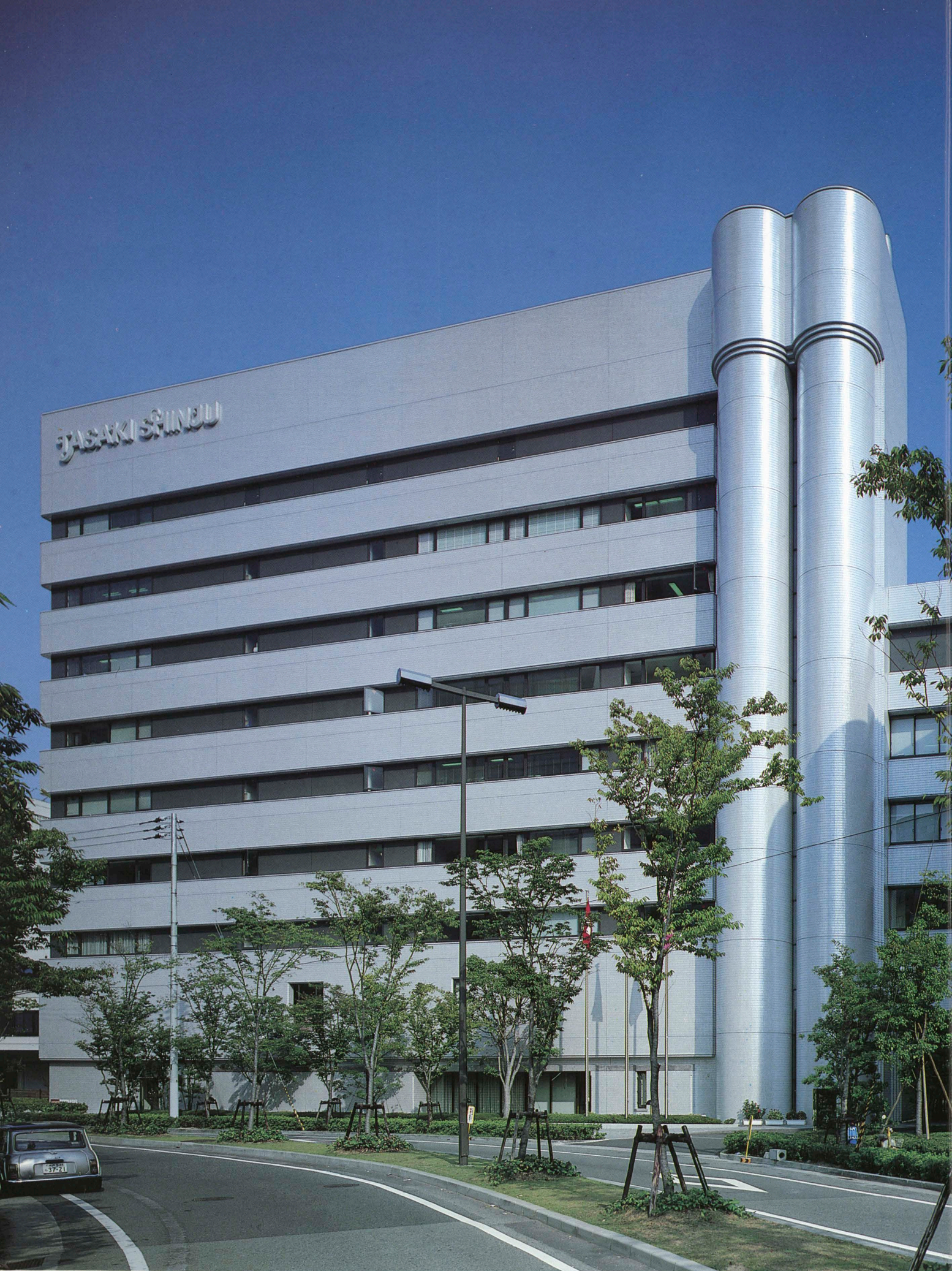
南東面全景 South-east side.
