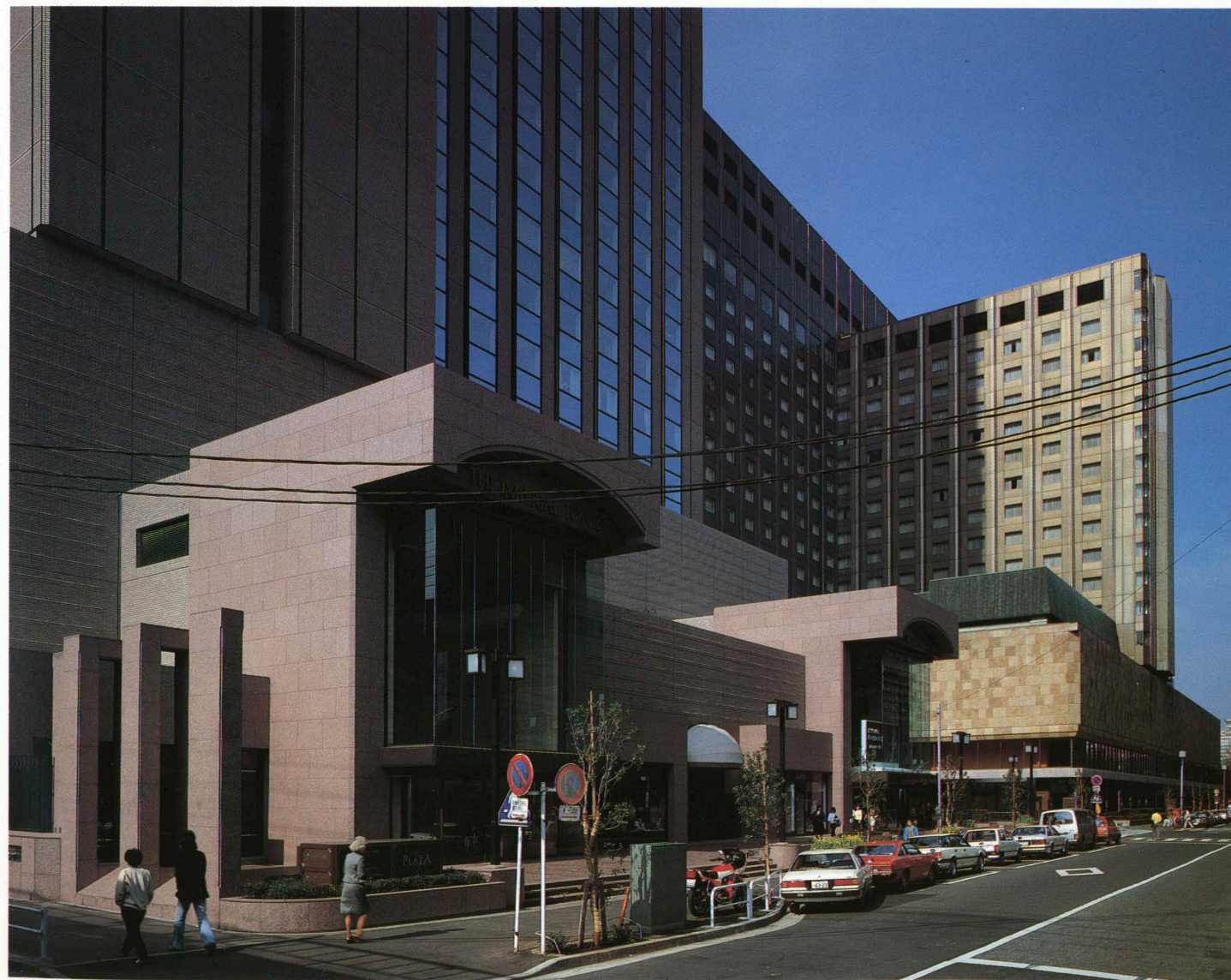
正面入口廻り外観 右は西側よりみあげる (above) Front side. (right) Upward view of the west side.
