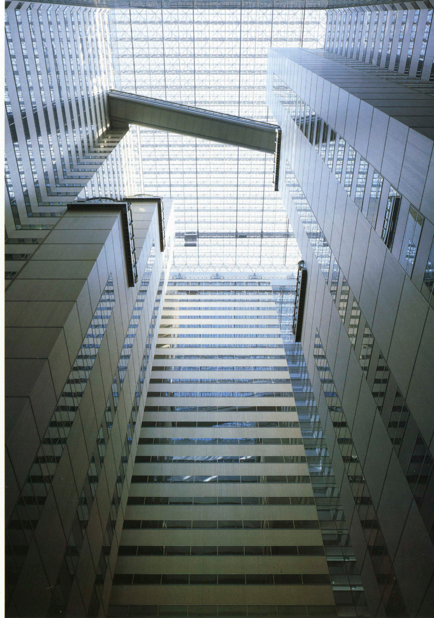
中庭をみあげる 左は中庭のみおろし (above) Upward view of the light shaft. (left) Downward view of the light shaft.
