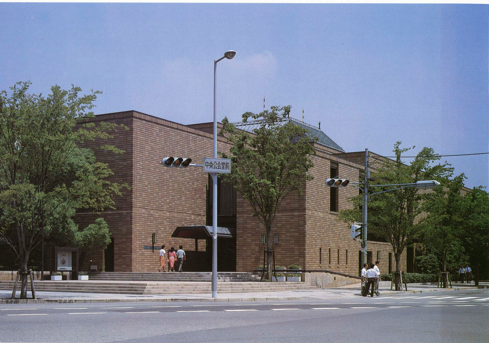
西側正面外観 General view of the front side.
