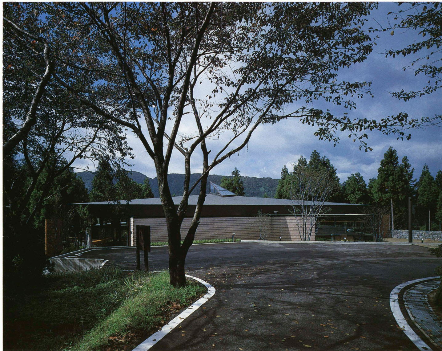
東側外観 右は南側外観 (above) East side. (right) South side.
