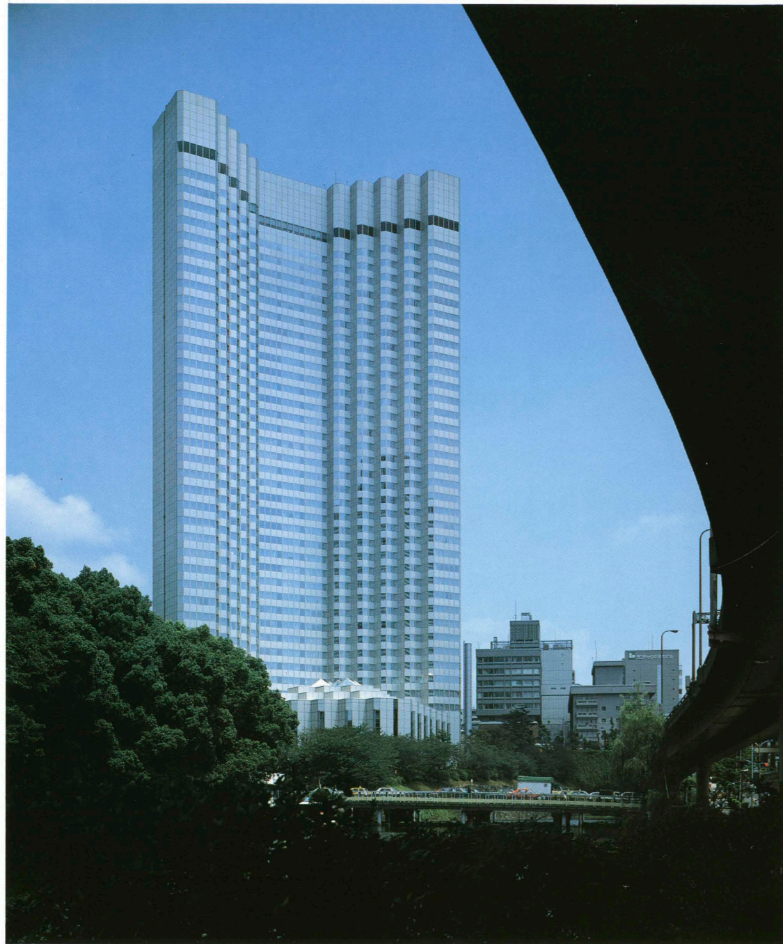
弁慶橋越しにみた全景 General view from the west.
