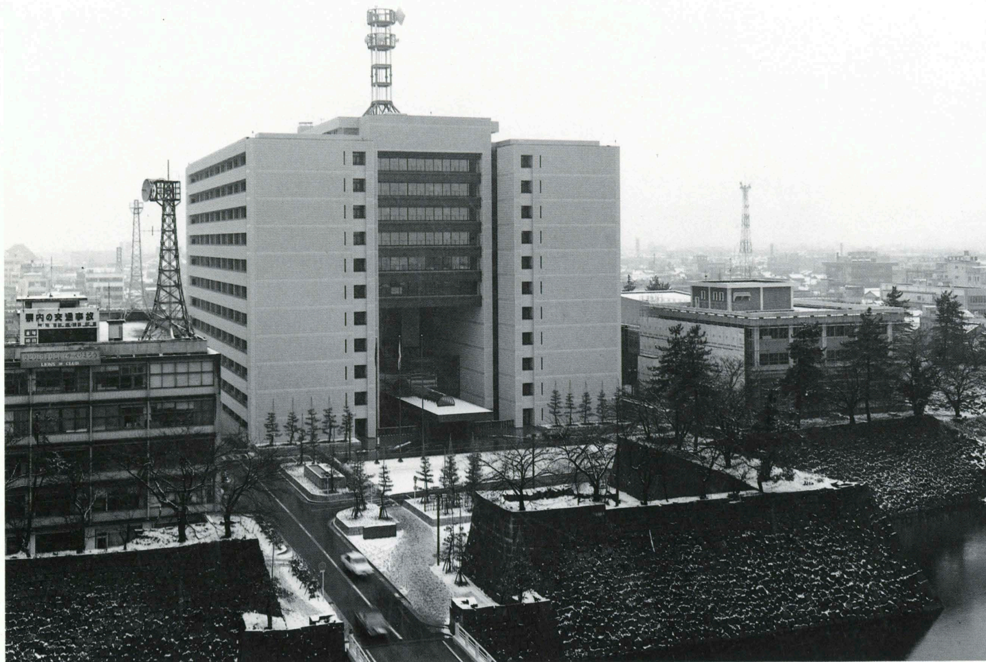
南側全景／General view of the south
