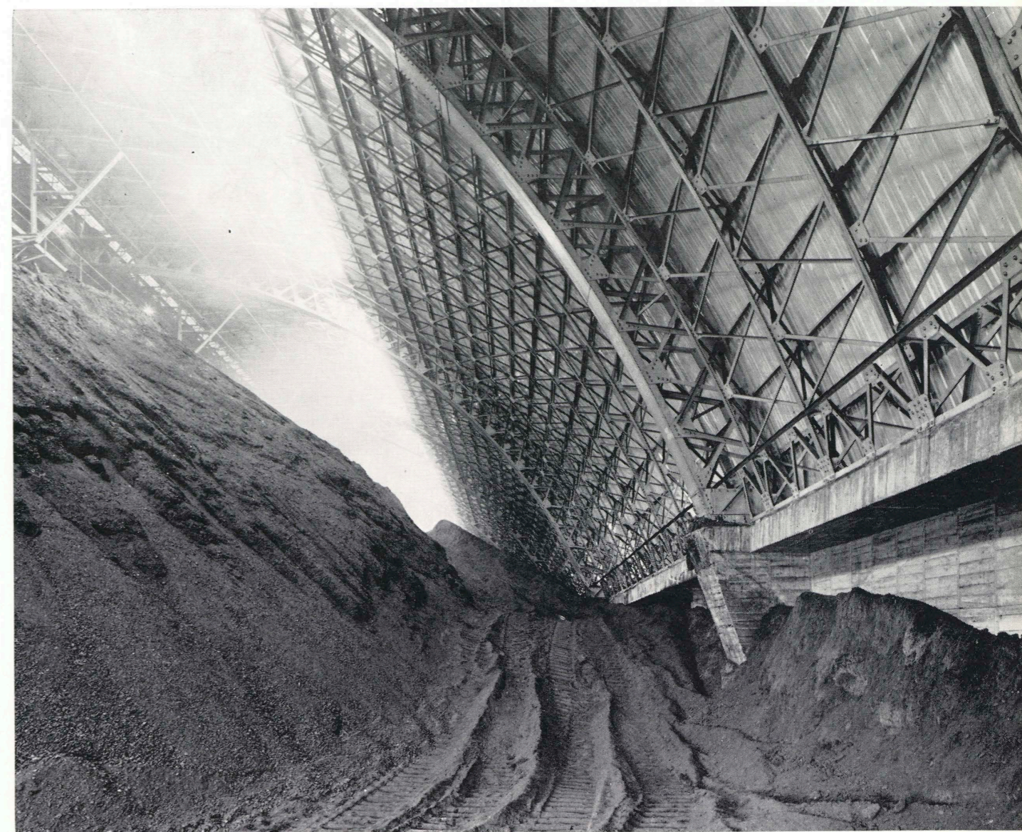
貯炭所内部 inside view of coal storage
