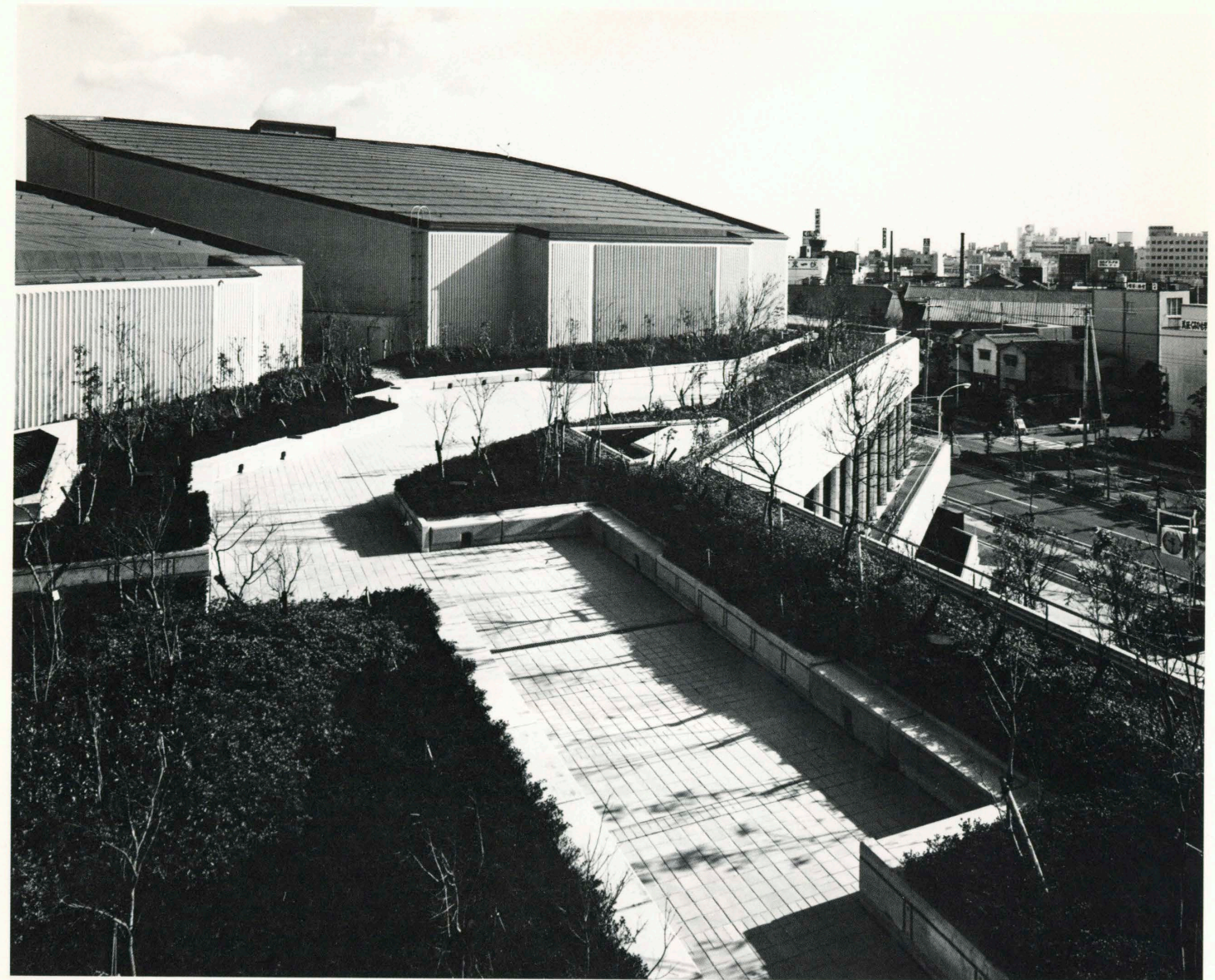
屋上庭園, Roof garden.
