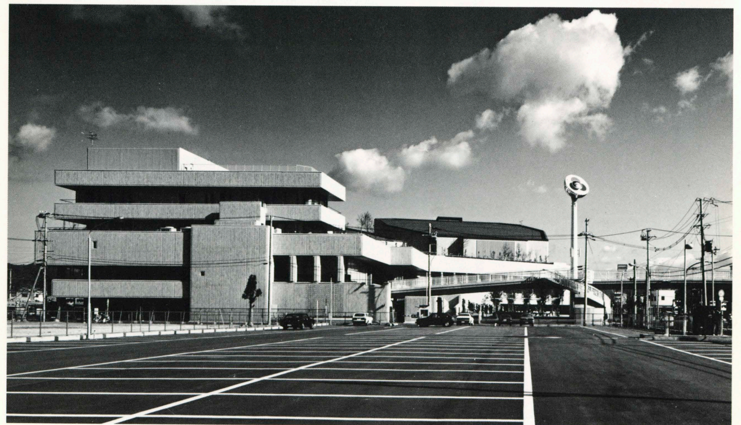
南西よりみる, 会議・練習棟, View of the conference hall from the southwest.
