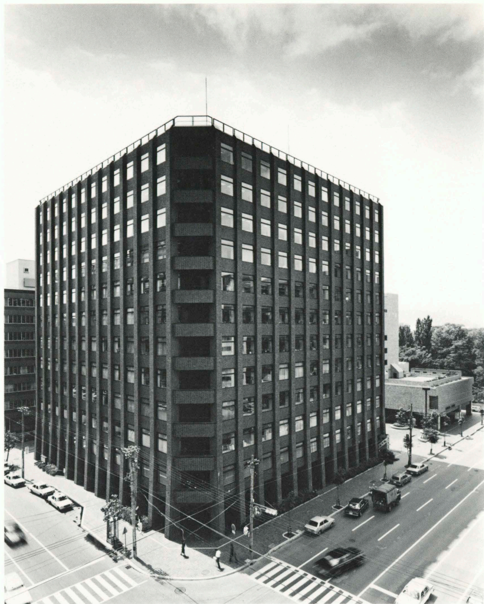
北東より業務棟をみる. View of the office wing from the northeast.
