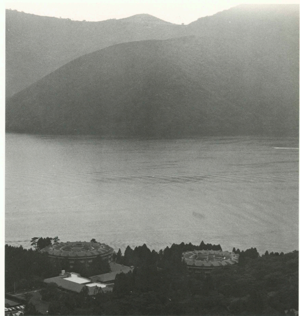
東より望む View from the east.
