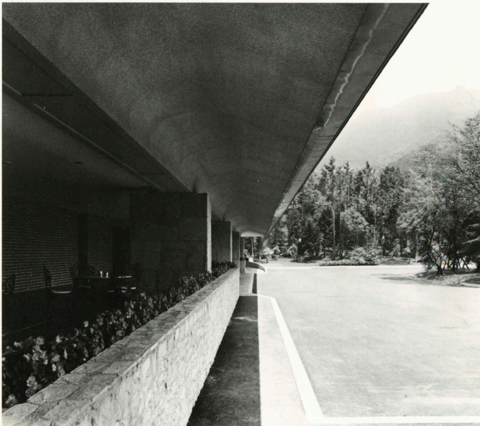
玄関の庇 Entrance eaves.
