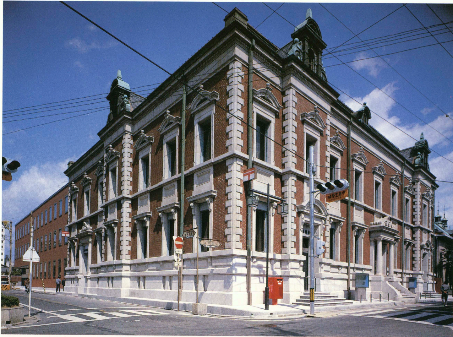
全景 (手前が外壁保存部分, 左奥が新築部分) General view. (the restored outer shell of the old building (right) and the new building (left).)
