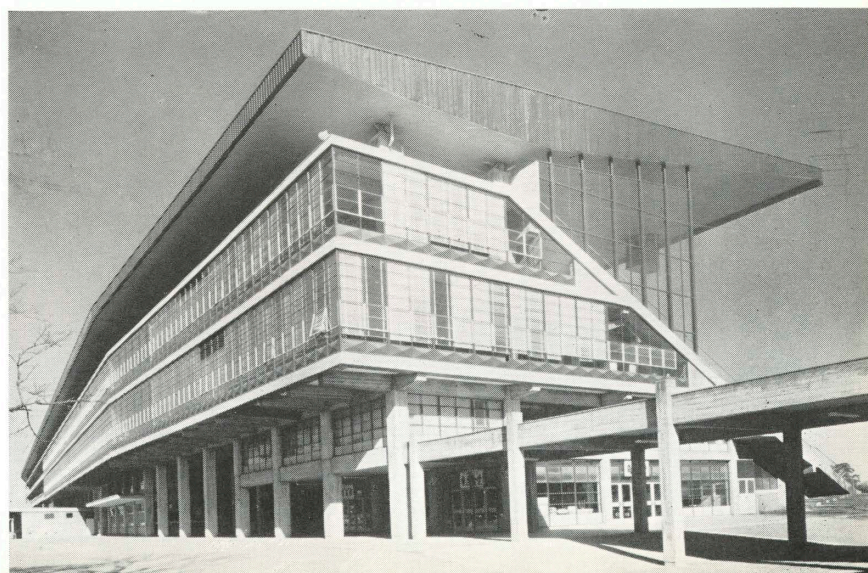
南門渡廊下側より connecting corridor of south gate
