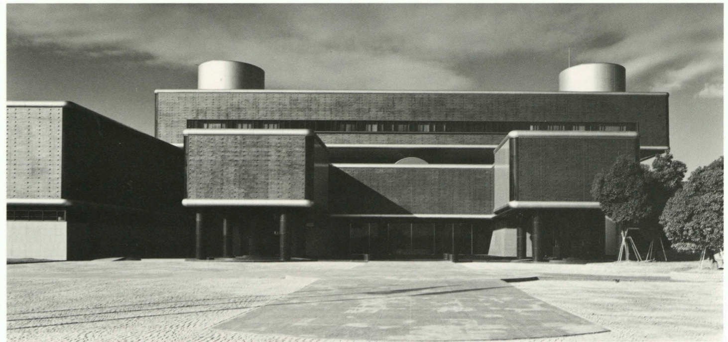
東側正面外観 Outside view from the east.
