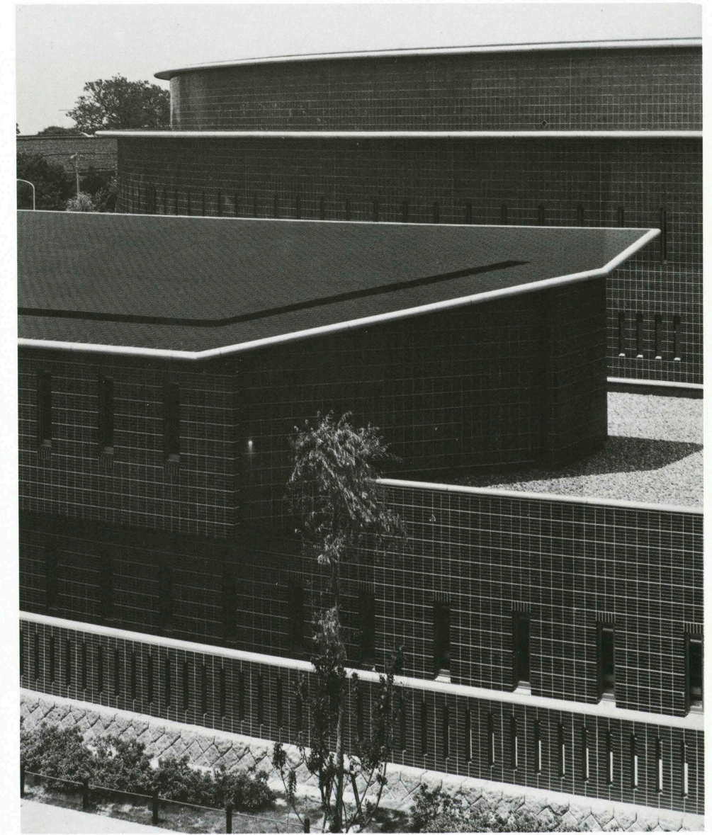
東側外観 View from the east.
