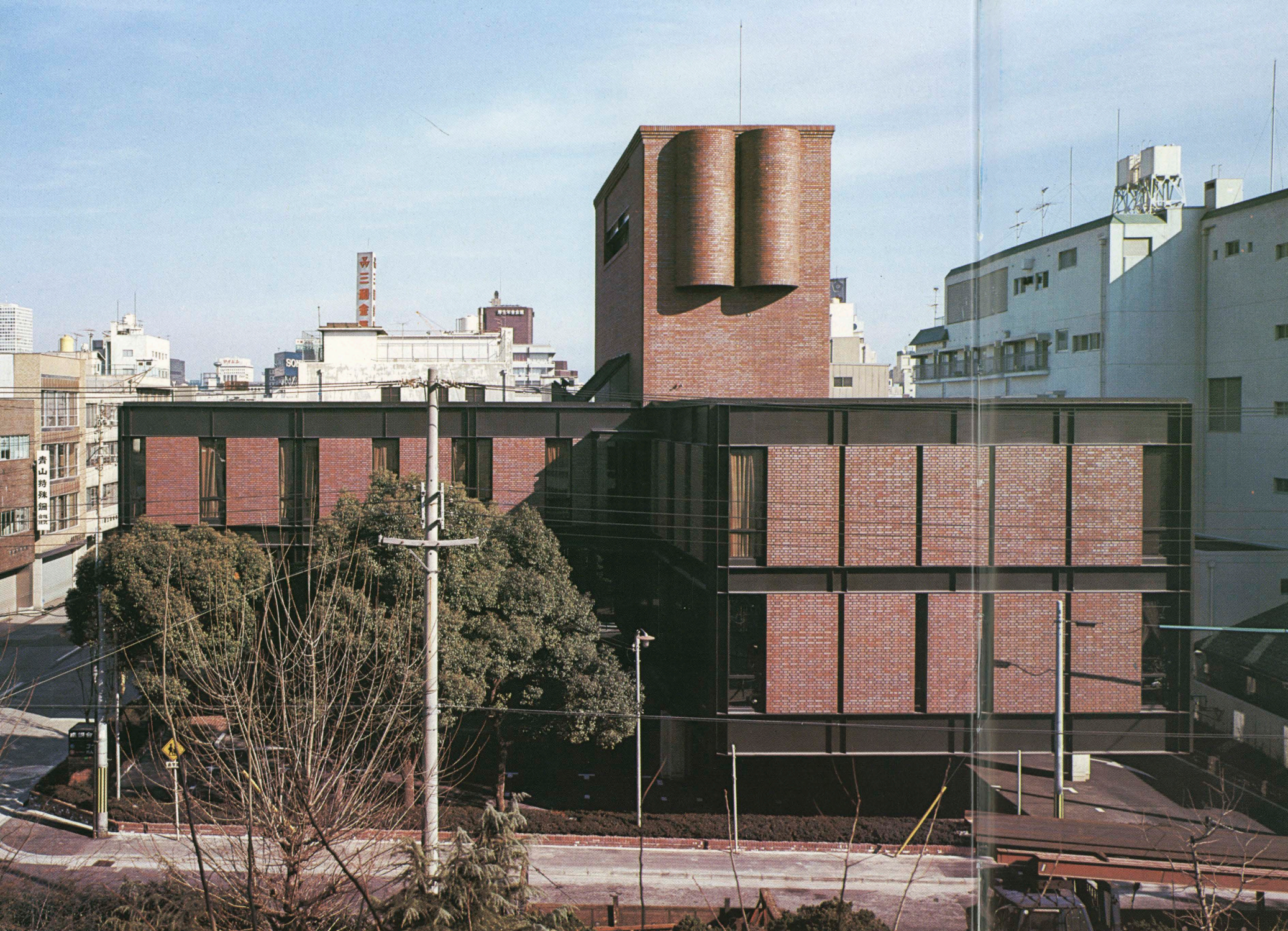
西側全景 General view from the west
