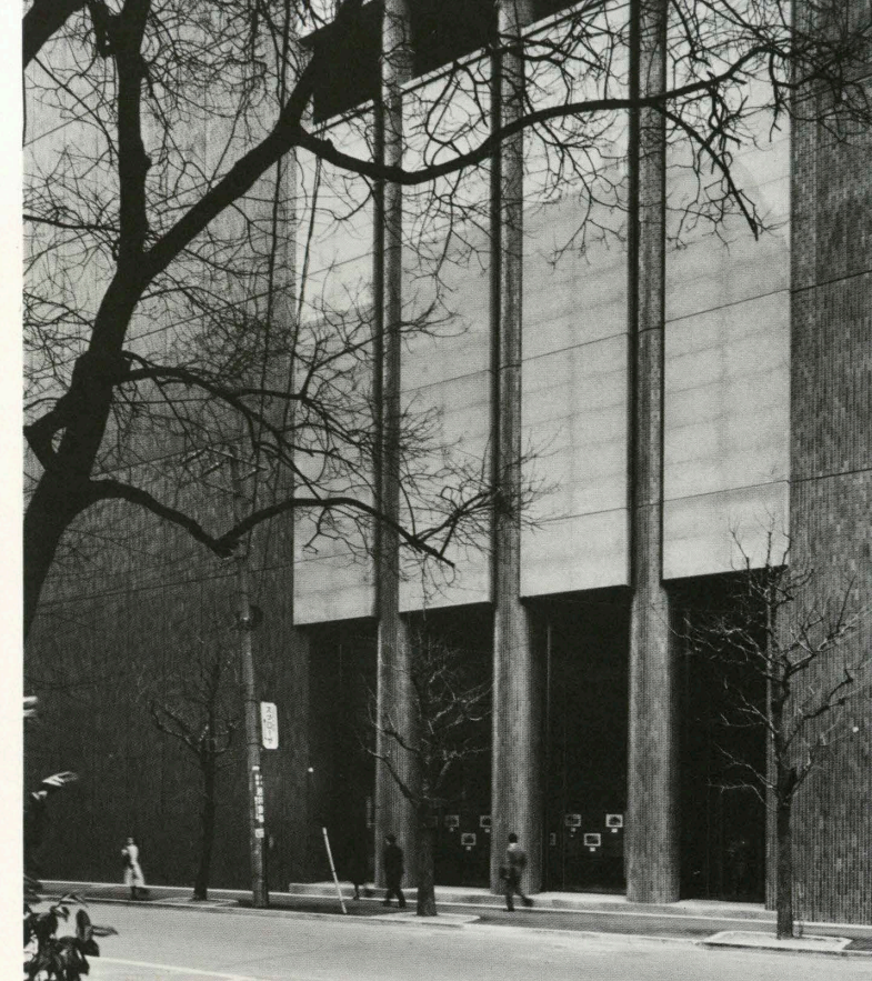
北側ファサード／North-side facade
