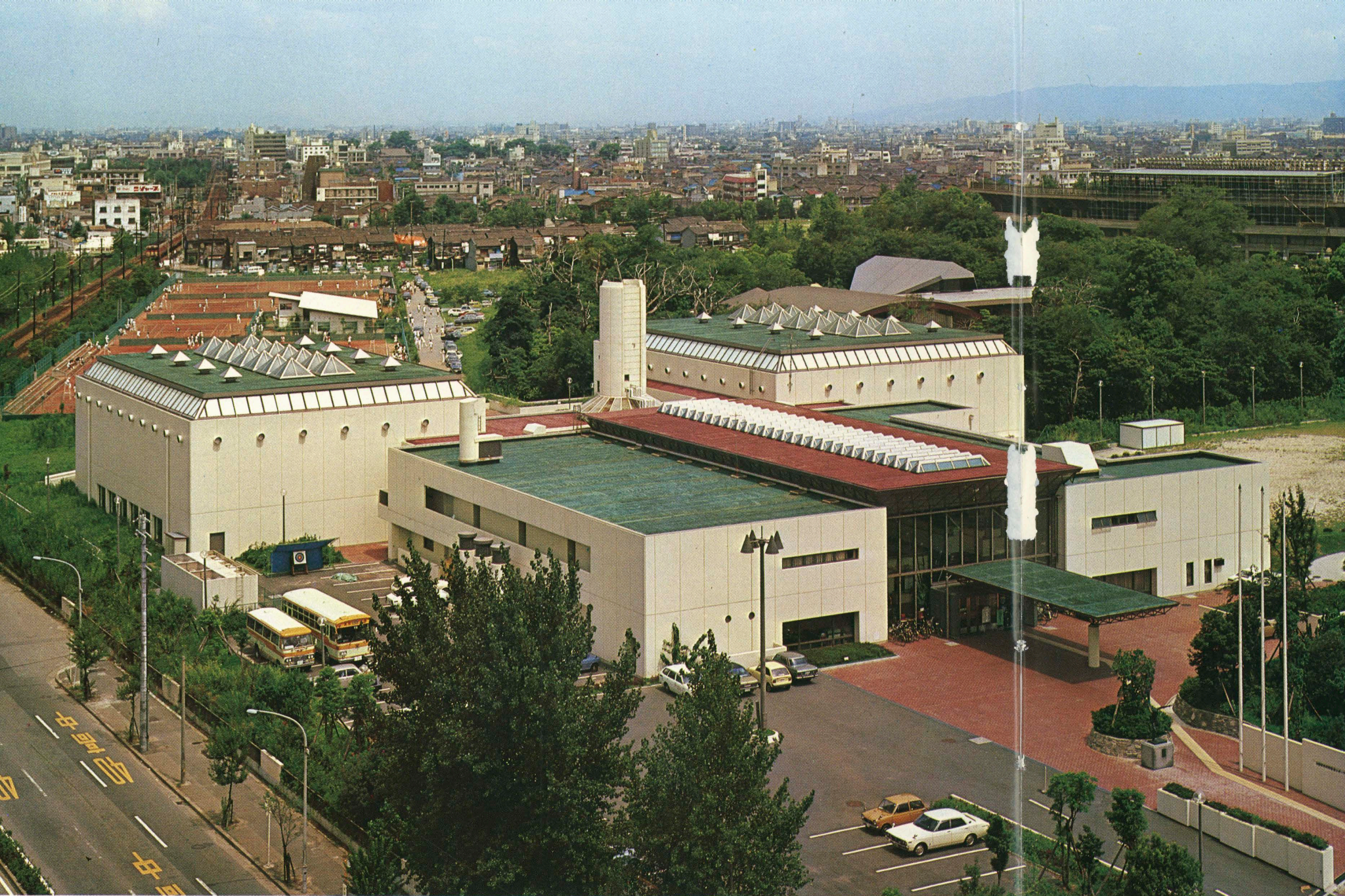
南西よりみる View from the southwest.
