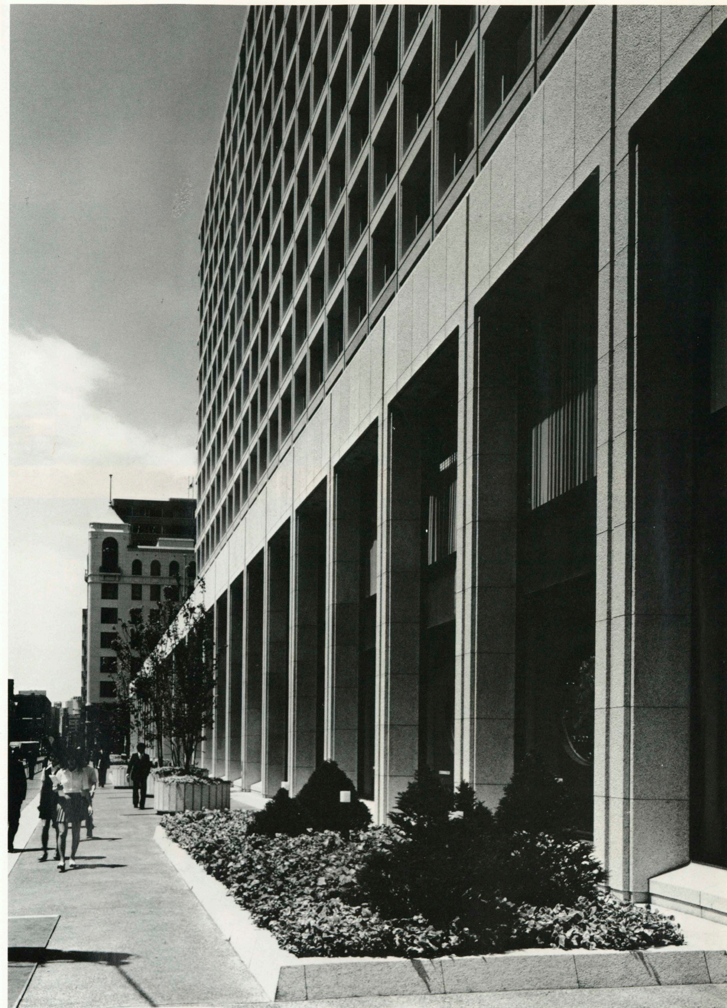
正面外観 Part of the exterior
