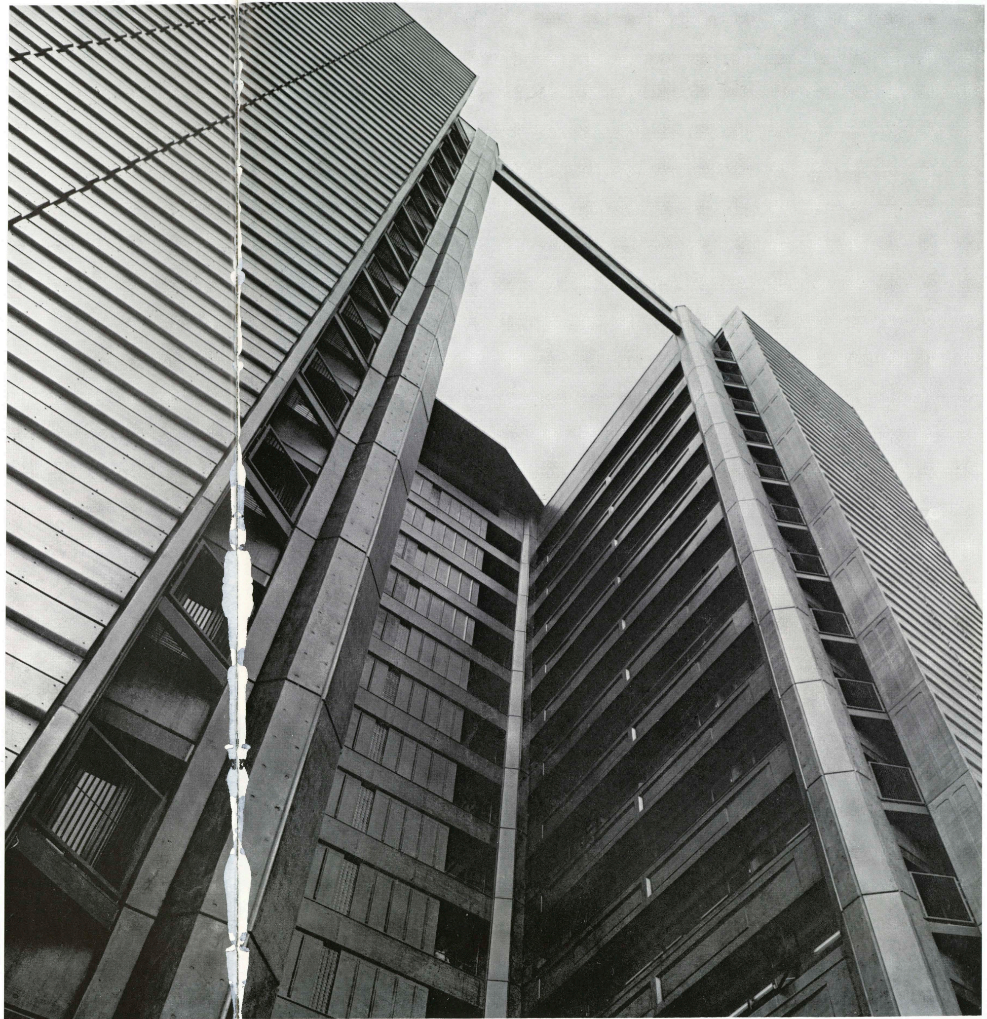
外觀部分 Exterior looked up from the main entrance
