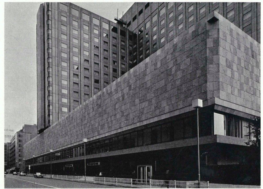
北面外観 North side exterior
