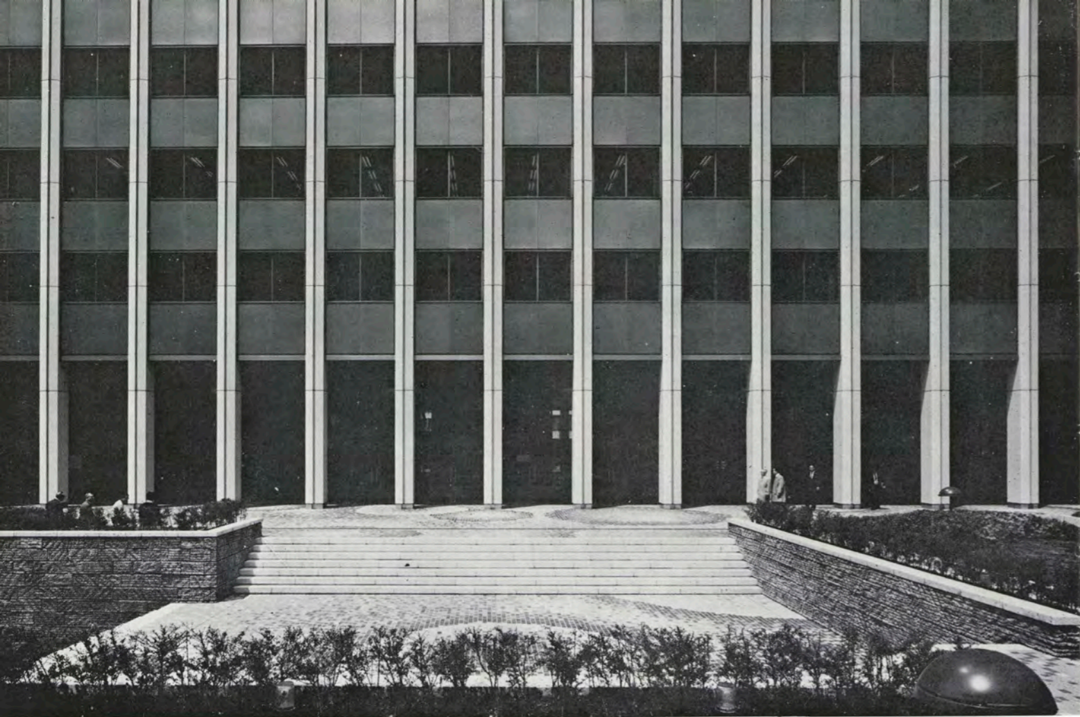
東南側外観 Southeast Exterior
