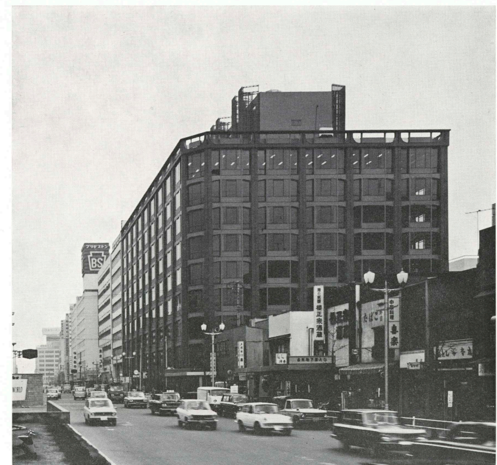
西北側全景 General View on the Northwest
