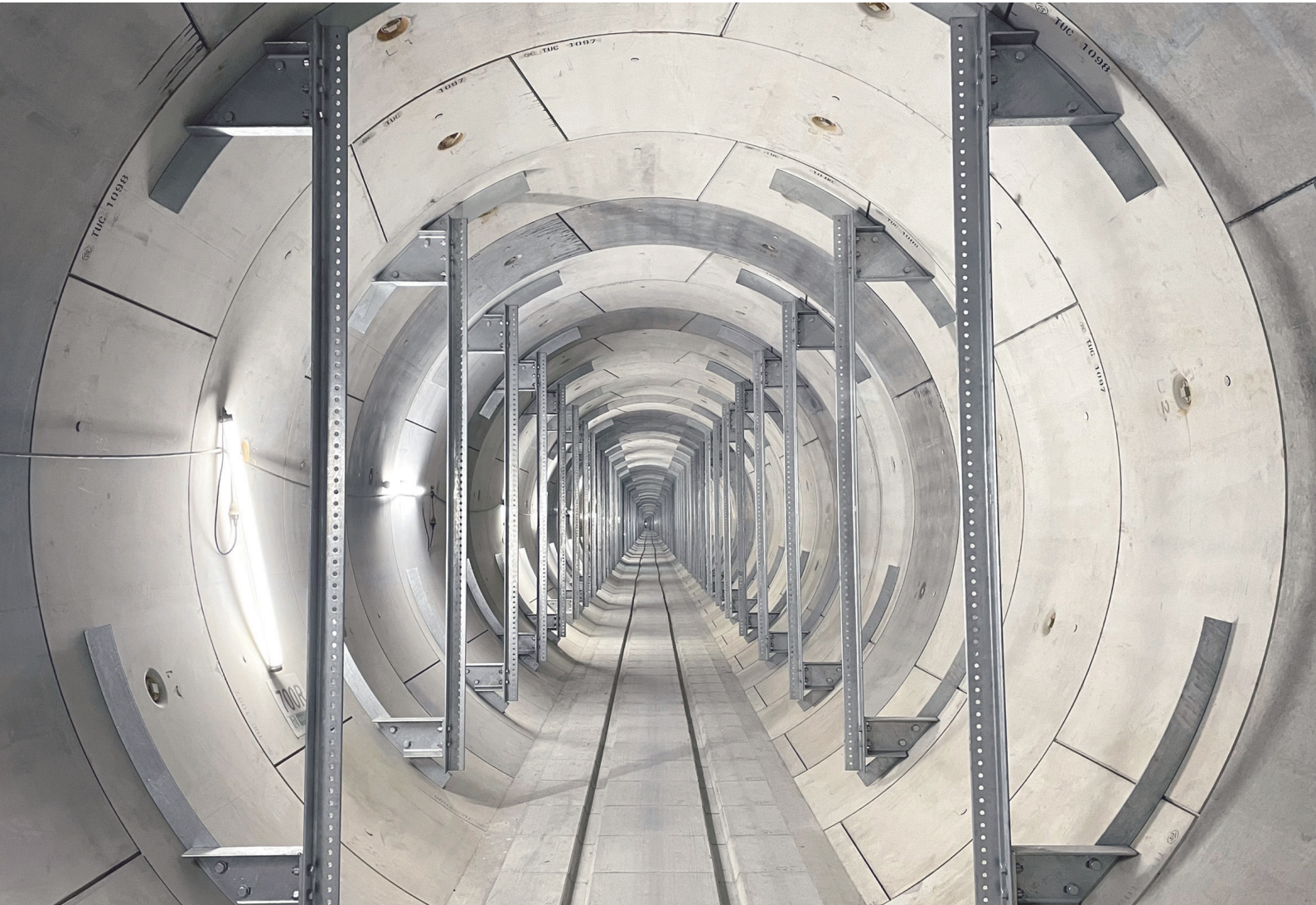
坑内完成状況 Inside of finished tunnel
