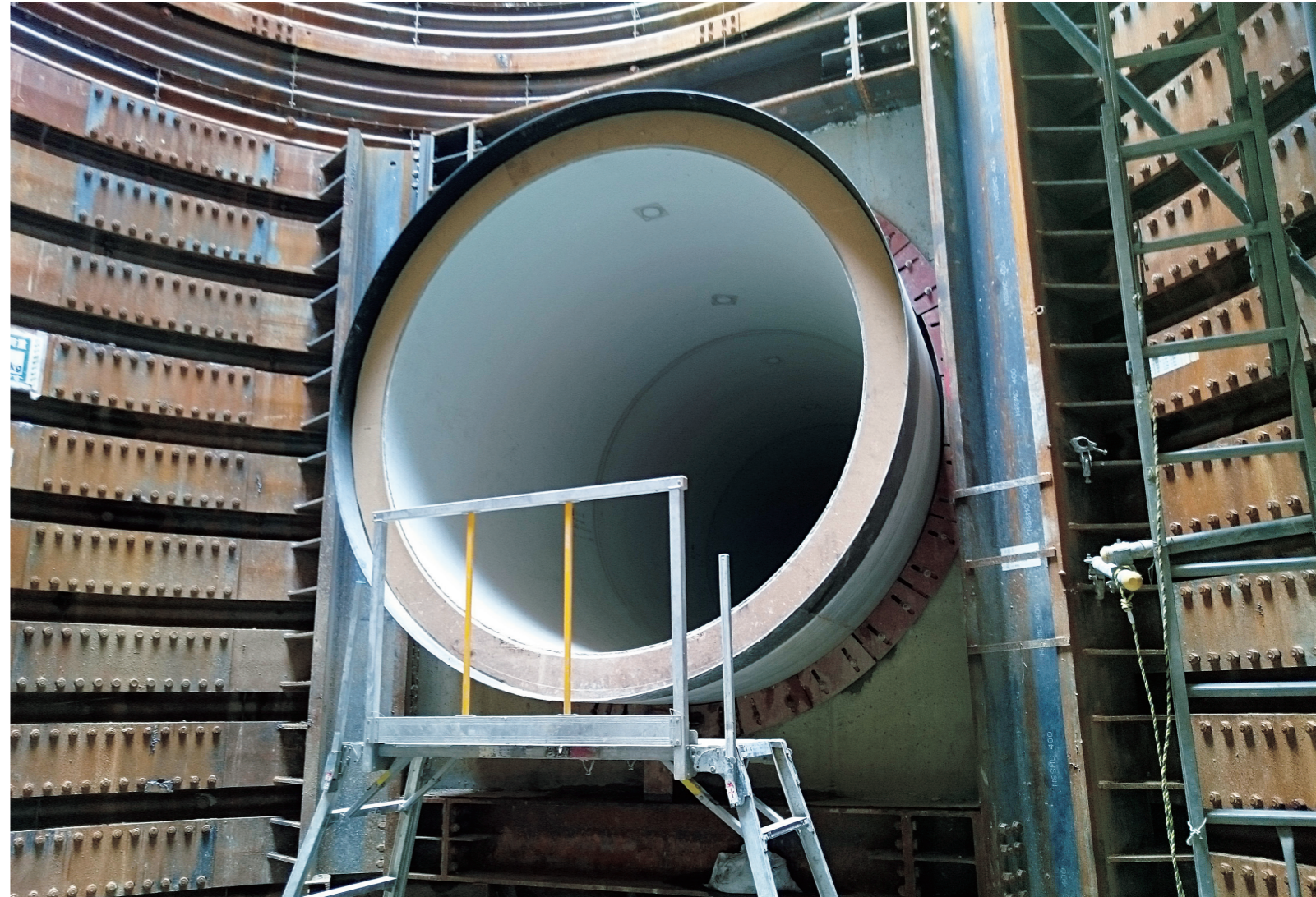
移設管の発進側 Starter shaft of the conveyance tunnel
