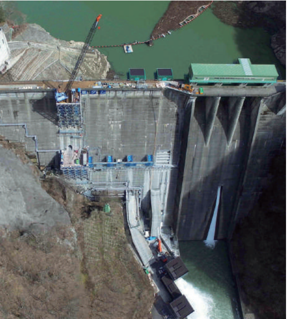
堤体の削孔施工状況 Drilling of the dam body
