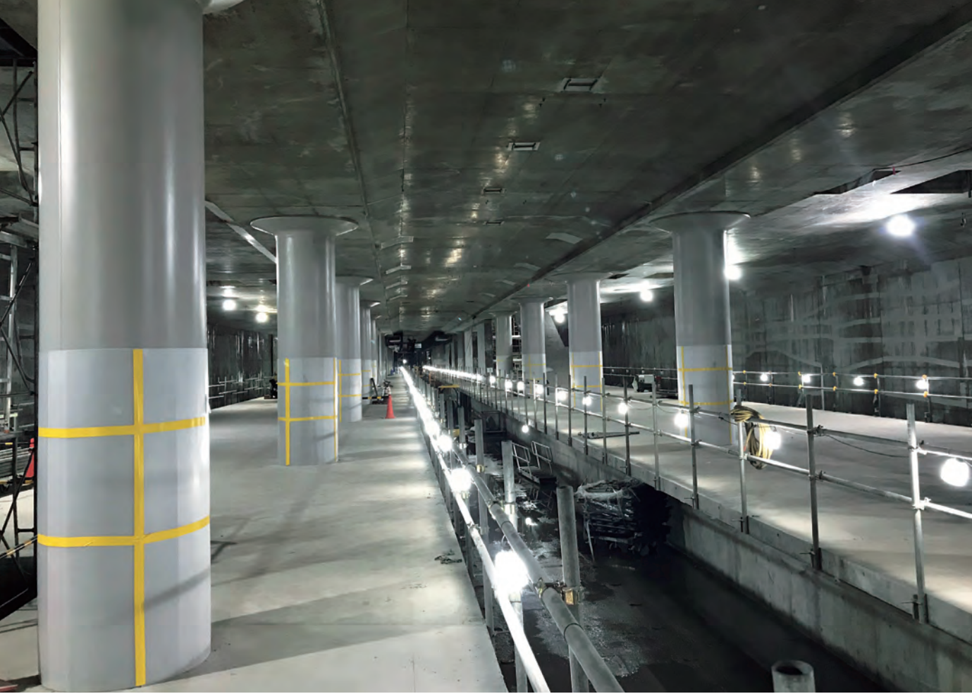
地下4階の相鉄東急直通線の躯体竣工時 Completed station structure of the Sotetsu-Tokyu Link Line at the fourth basement floor level
