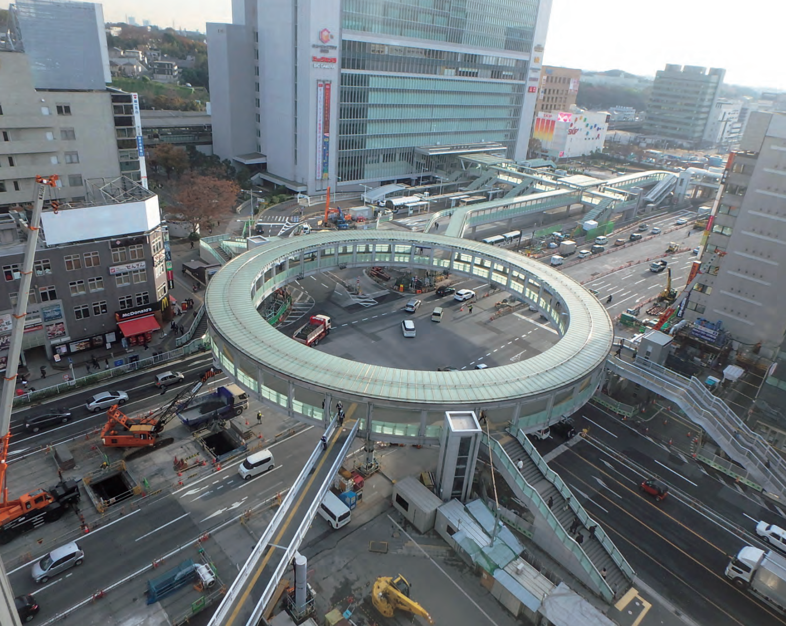
地上部の全景 Aboveground view of the station area
