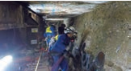
切羽掘削状況 Drilling status of cutting face
