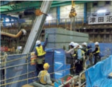
立坑掘削(上)、鋼製セグメント函体組立(下2点) Shaft drilling (top), steel segment box assembly (bottoms)
