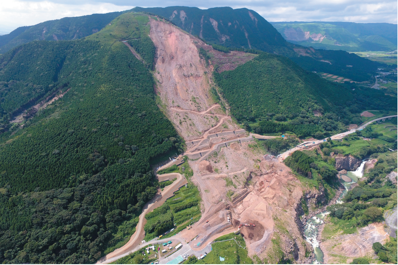
緊急対策工事完了 Completion of emergency measure construction
