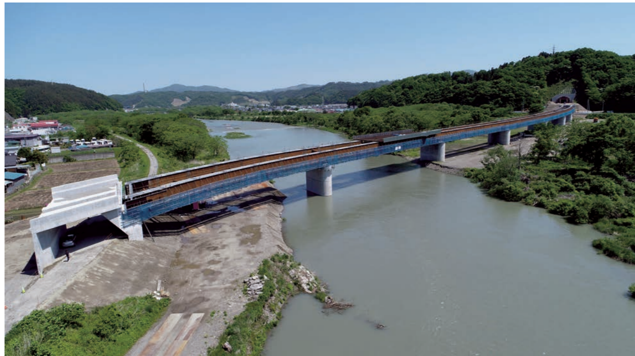
写真-1 (仮称)閉伊川横断橋
